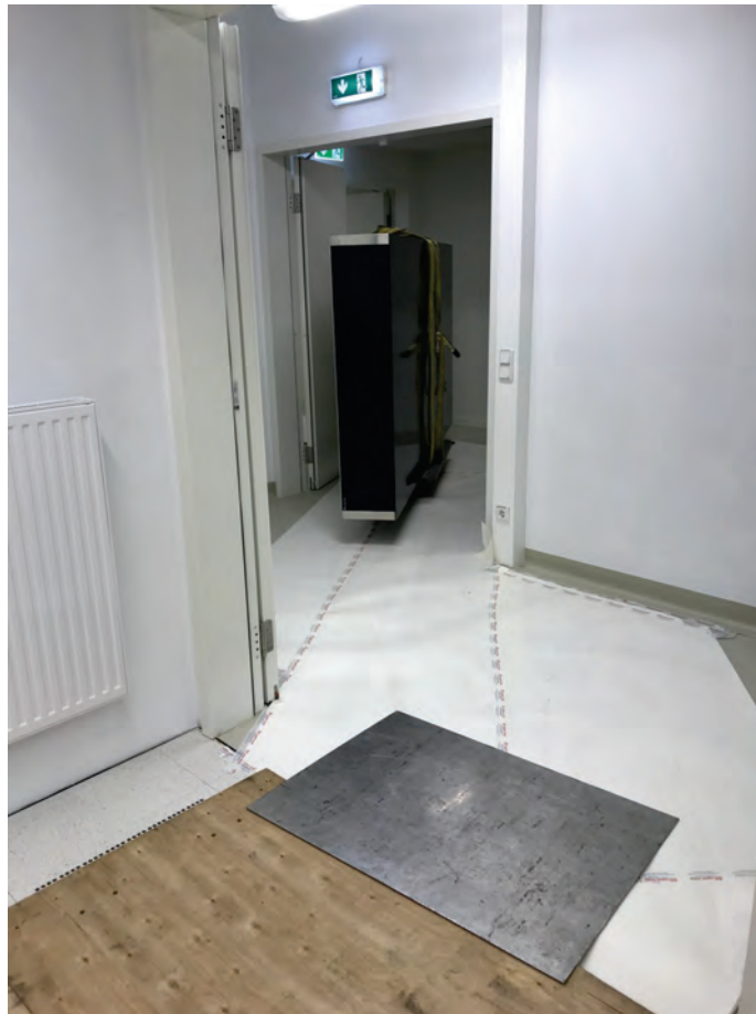
Fig. 4: Moving an optical top through the building; photo credit: TMC
