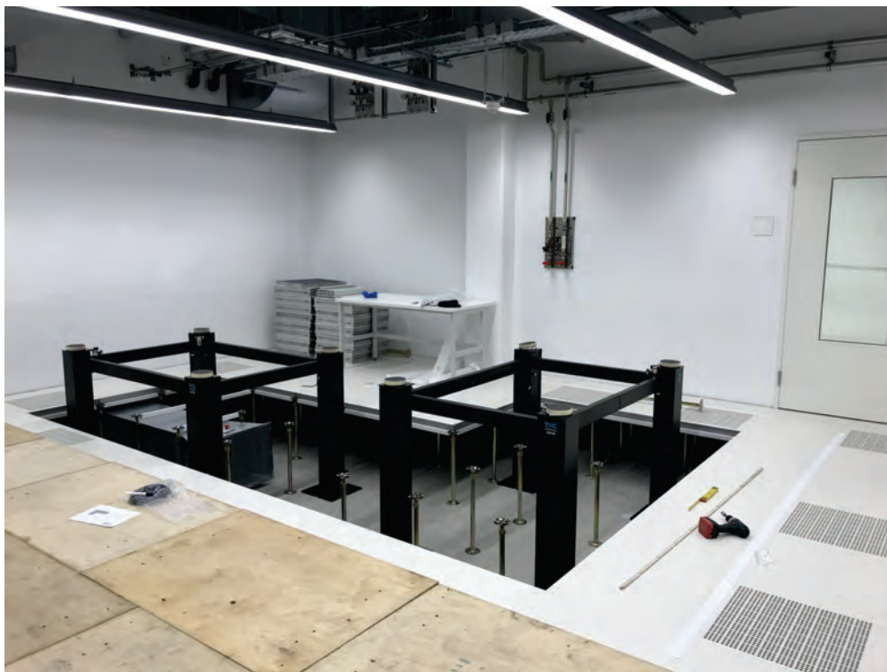
Fig. 8: Post Systems completed, base plates bolted to the concrete floor; photo credit: TMC
