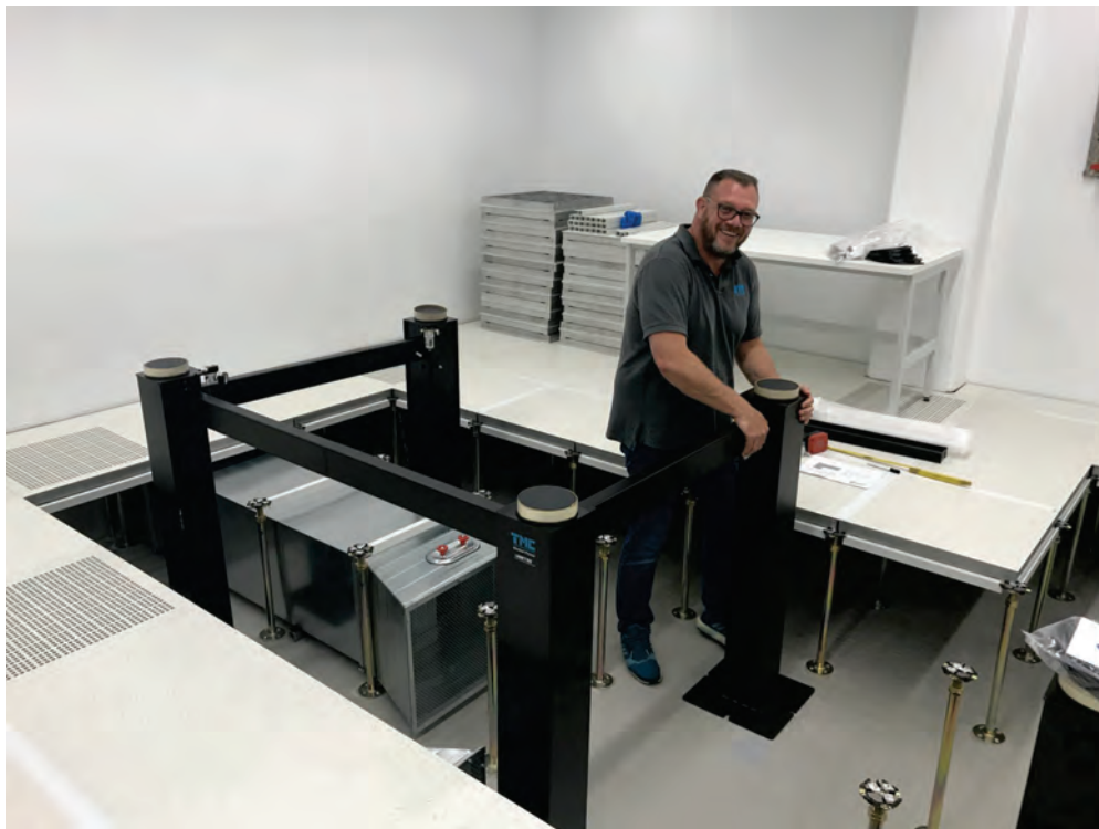
Fig. 7: Isolation of post systems inside raised floor; photo credit: TMC
